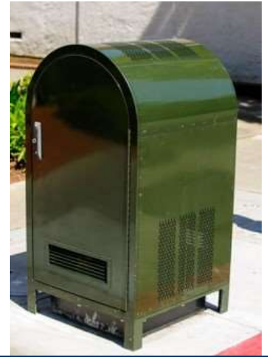
Not so “small” microcell disguised as a mailbox
